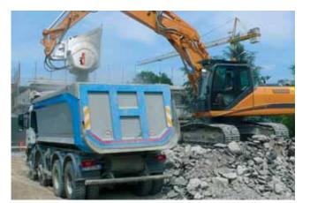
The rotor system can crush without problem the rebars.
